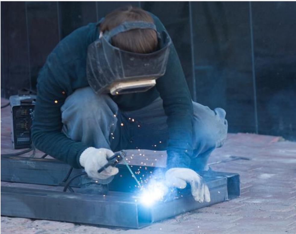
Welding on the floor
