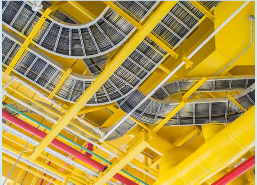
ABOVE: Cable trays, like the ones being made in this application, come in a wide variety of curves, lengths and widths to accommodate electrical cabling in industrial or residential applications.
