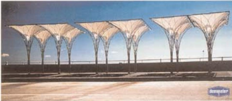
Fanning out, and up 14 ft to 8x8-ft frame, 0.625-in. stainless-steel rods from 6 x 42-in. base form structure of aesthetic light stanchions. Developed by Product & Design using the Demmeler modular fixturing system, they line the way at the Staten Island ferry terminal.
